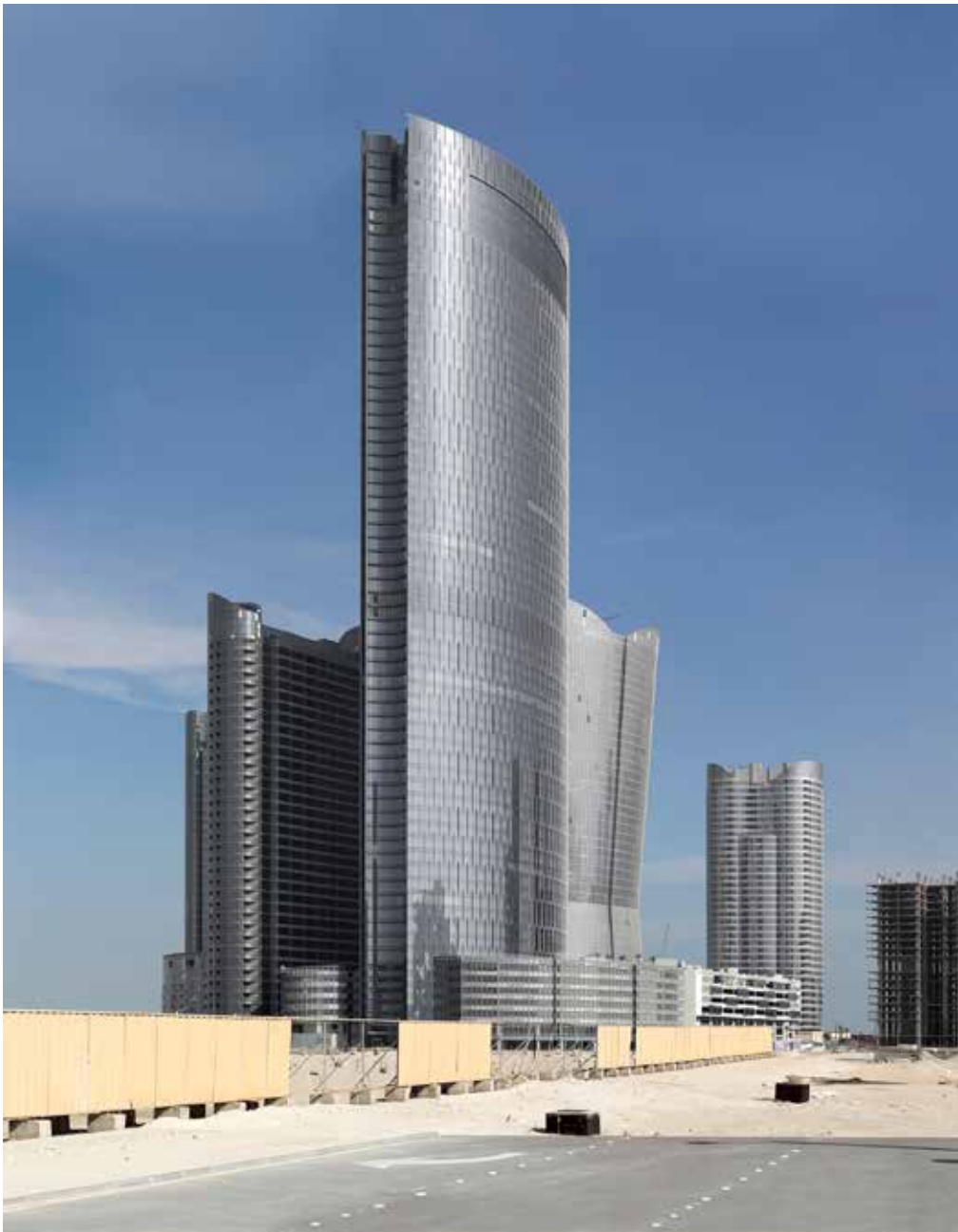
Construction Reem Island, Abu Dhabi, 2015
