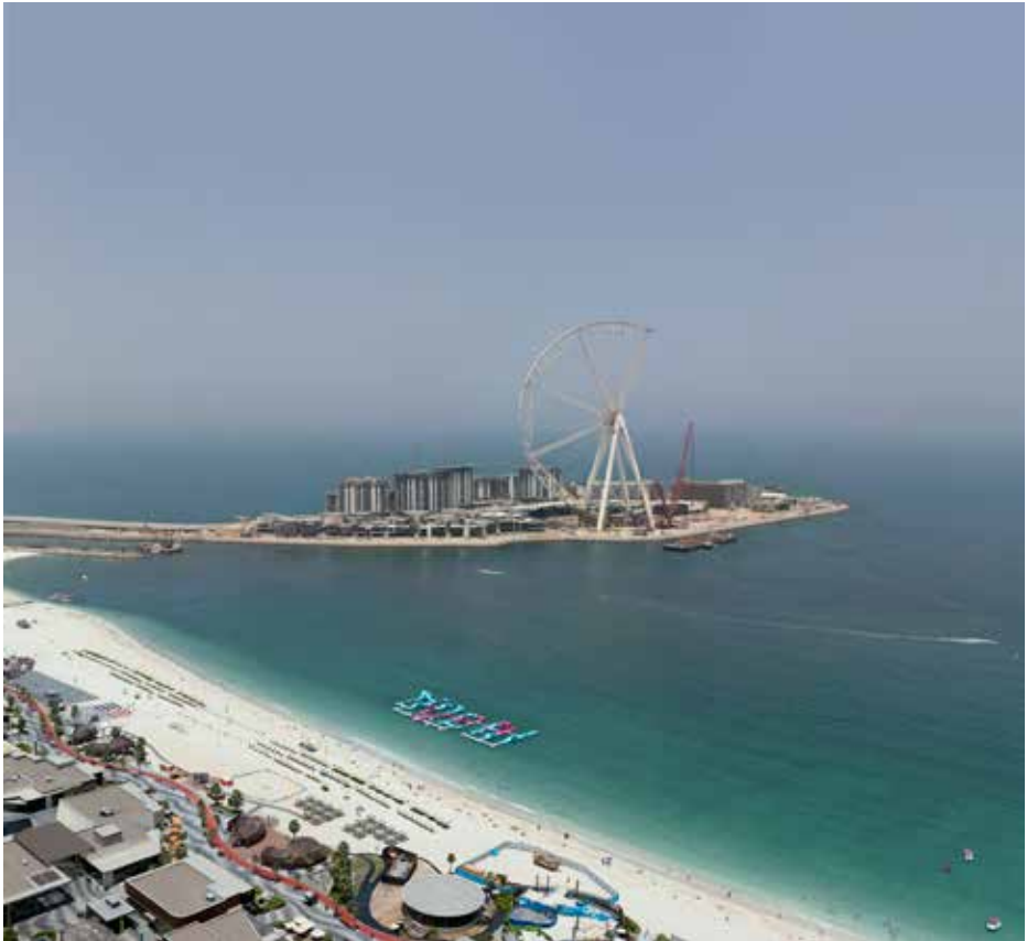
Construction of Giant Wheel Dubai Marina, 2017
